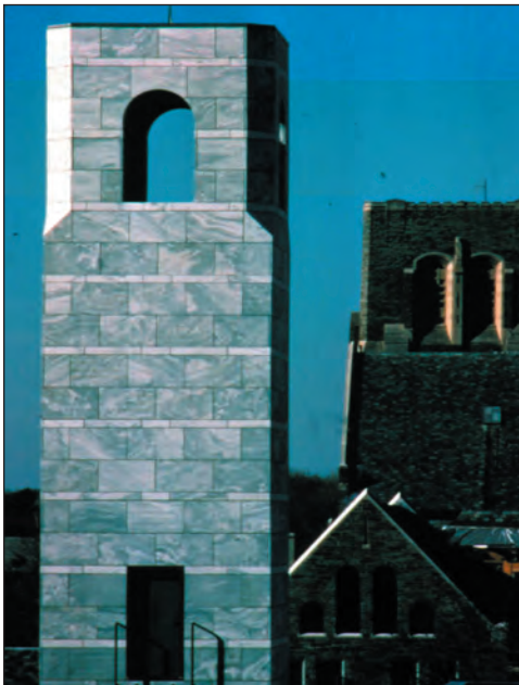
The tower on Schwartz Center for the Performing Arts is a modern interpretation of the Collegiate Gothic style as seen at Myron Taylor Hall in the background.
