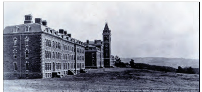
Stone Row from northwest, ca. 1871 -- The first buildings were placed on a site that had been treeless agricultural land.
