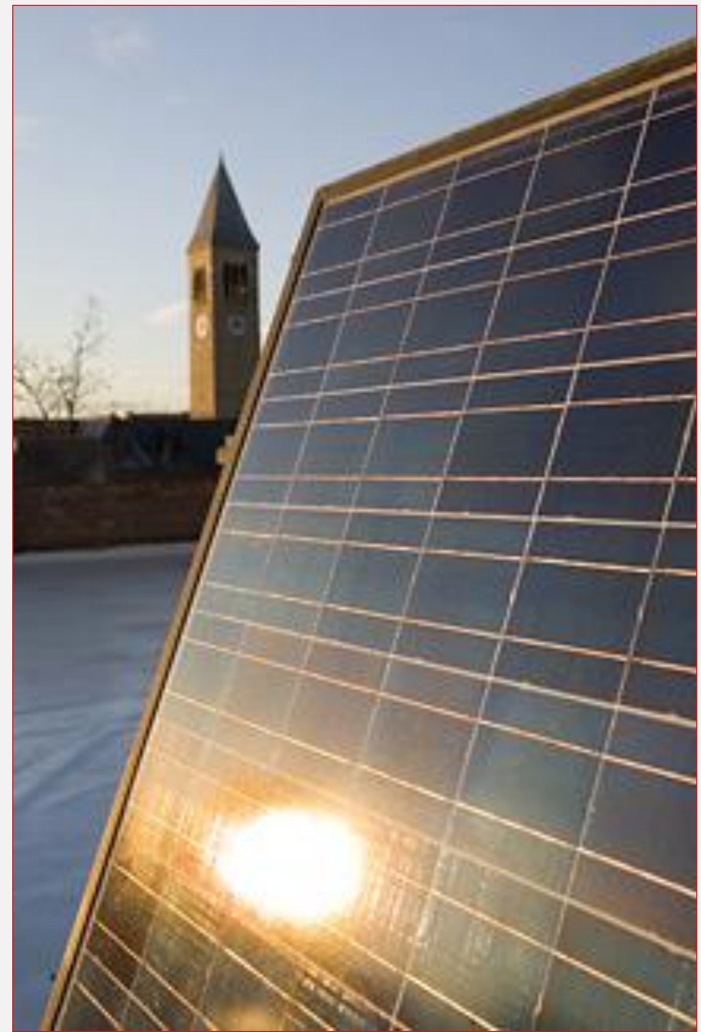
The Day Hall system powers the McGraw Clock Tower
