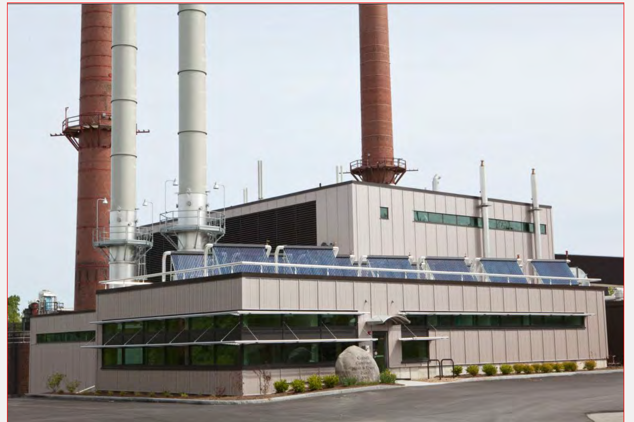
The Central Energy Plant Office Building
