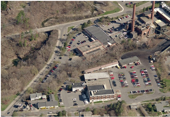
Humphreys-Maple Avenue Complex
